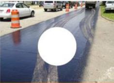
A liquid adhesive known as "tack coat" will be sprayed on the roadway ahead of the paving operation. Please avoid driving on or over the tack coat. It is a tar-based product that could potentially stain your driveway or vehicle. Caution should be used with pets and children, as freshly placed asphalt is extremely hot. Please follow instructions from on-site workers.
